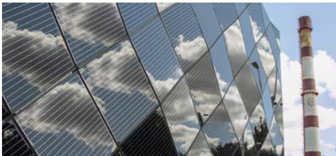
Figure 3: Solar panels at cooling station in Tartu
