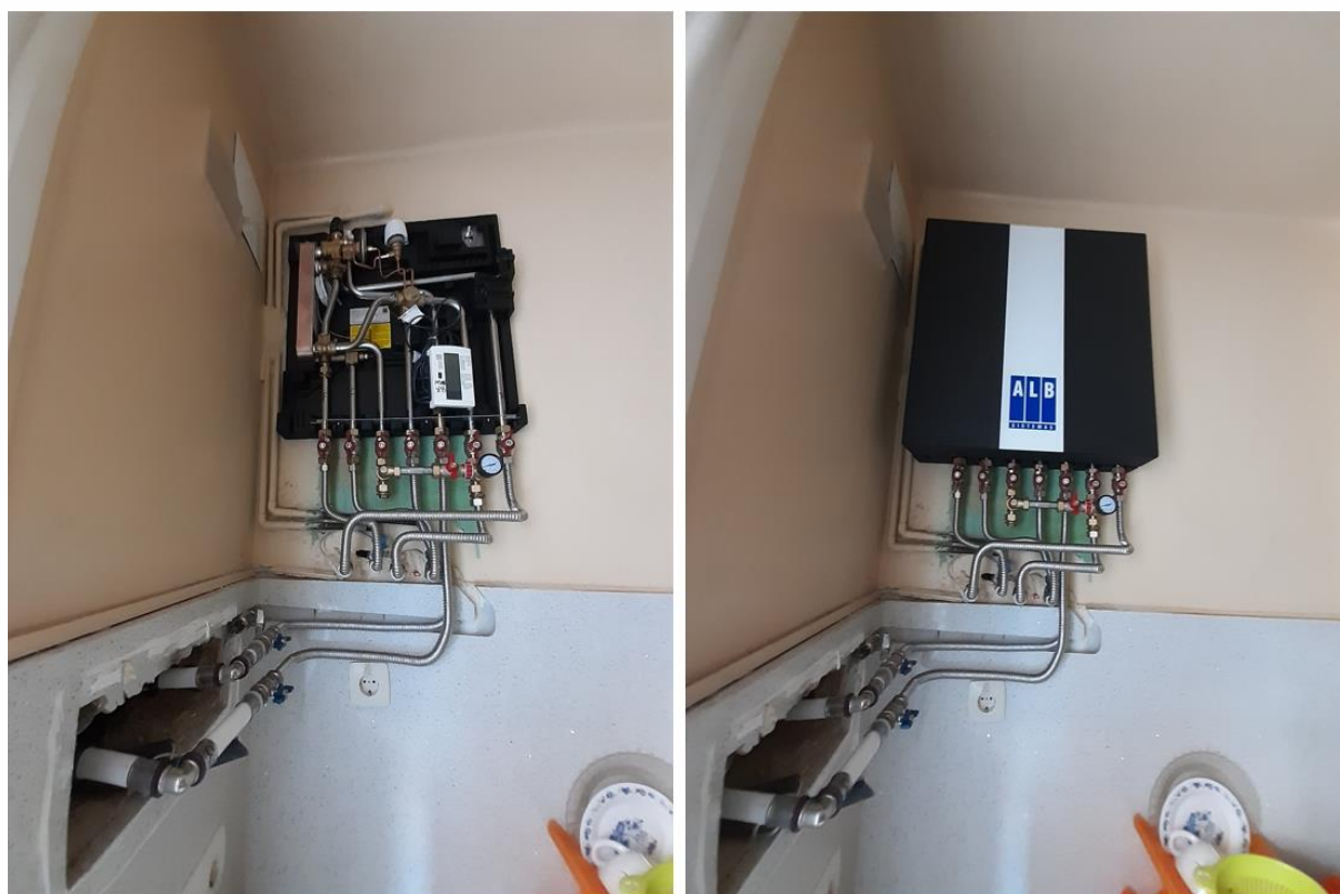
Figure 26: District Heating Network. Dwelling's individual heat exchanger. Open and closed. (source VIS)
