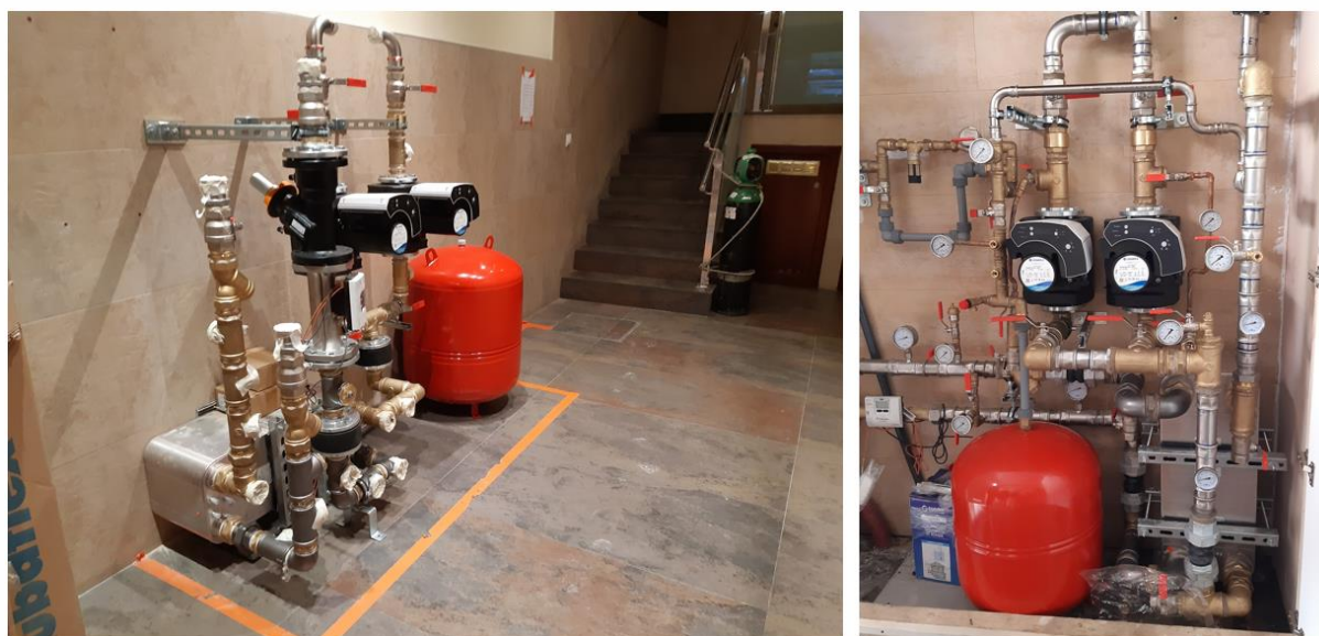
Figure 25: District Heating Network. Building's substation (source VIS).
