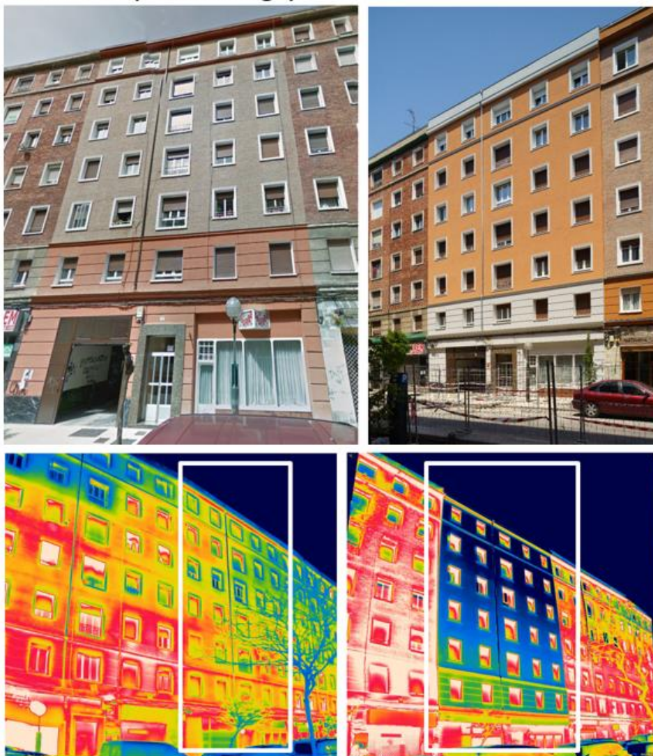
Figure 30: Badaia 8. Thermal scan. Before & after (source VIS)
