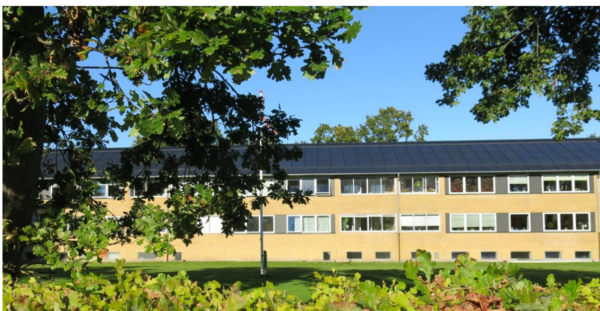
Picture 23 Roof-top integrated PV panels dept. 11 Sobo
