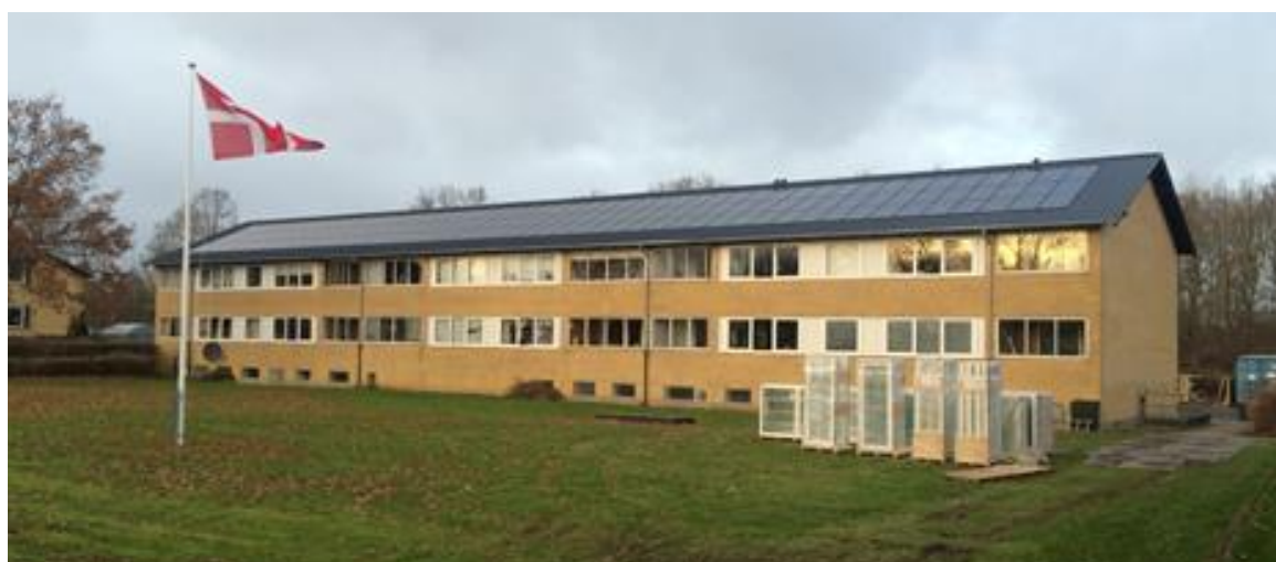
Figure 2: SOBO Department 11, Building integrated solar cells
