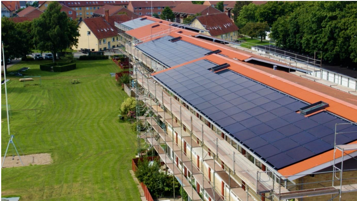
Figure 12: SAB Department 18, 730 m2 solar PV panels integrated in the roof combined with 75 kWh battery capacity
