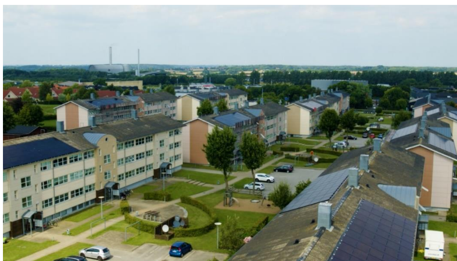
Figure 11: SAB department 24, 1,870 m 2 solar PV panels integrated in roof combined with 200 kWh battery capacity. Each of the 10 buildings has one solar PV panel-system and a battery in the basement. Department 24 has 324 apartments.
