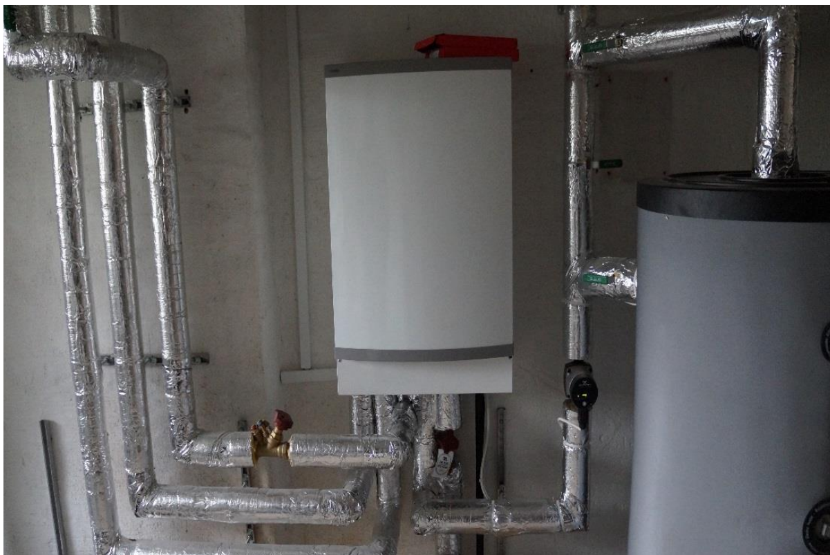
Figure 3: SOBO Department 11: New heat exchangers for district heating
