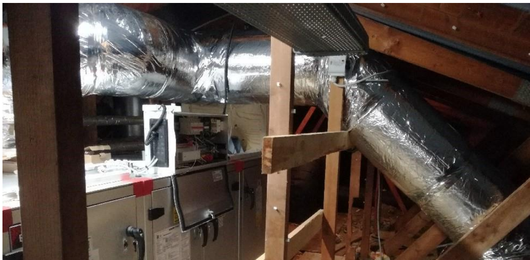
Figure 10: B42 Department 21: New ventilation system with heat recovery
