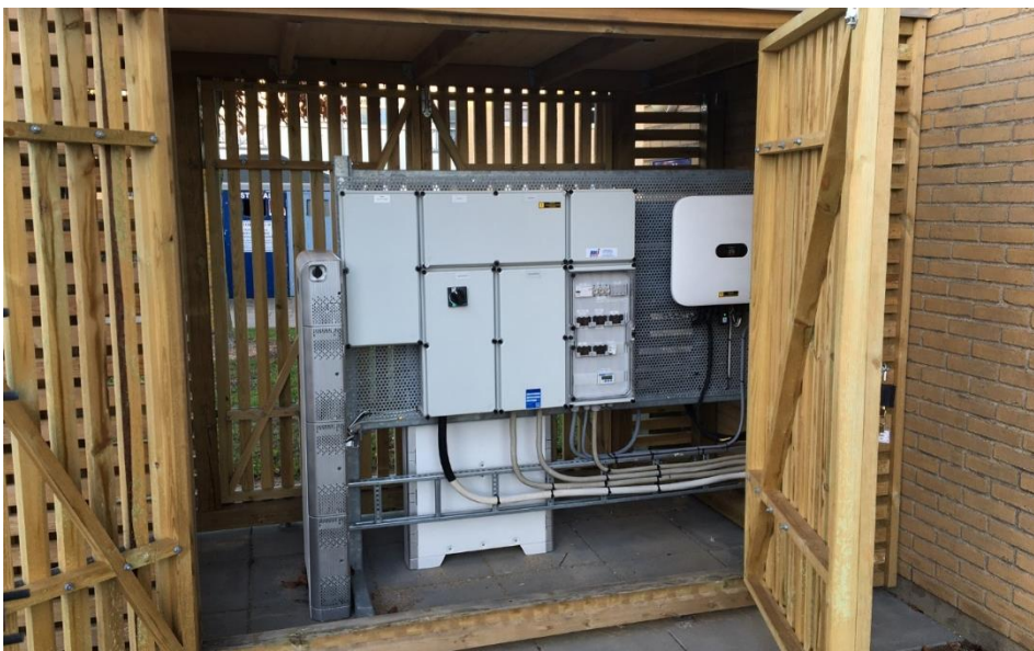
Figure 13: SAB Department 21, The batteries are installed in technical rooms outside the buildings
