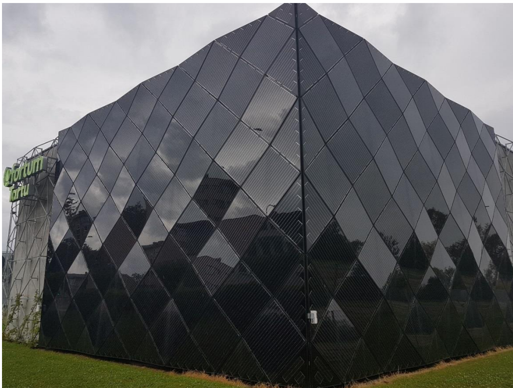
Figure 4: Facade of cooling plant with solar panels
