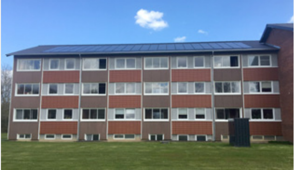
Retrofitted housing association building with roof integrated solar panels and battery storage solution. Credits@ProjectZero.
