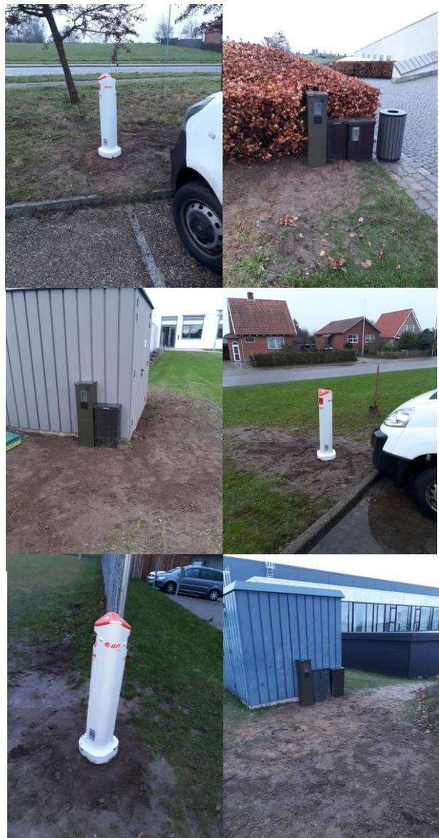
Figure 6: Installed public chargers and metering units
