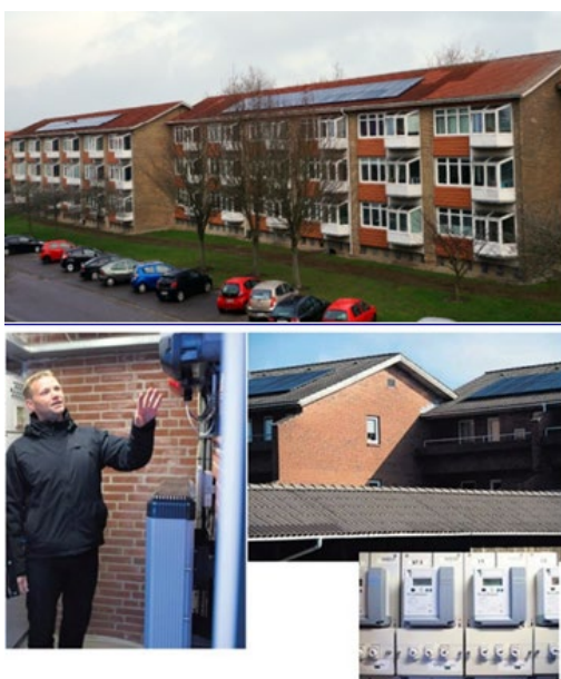
Pictures: PV-panels and energy storage scheme on renovated buildings in Sonderborg. Credits: Sonderborg Municipality.
